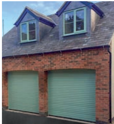
Garage under a bedroom?
